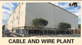
CABLE AND WIRE PLANT
